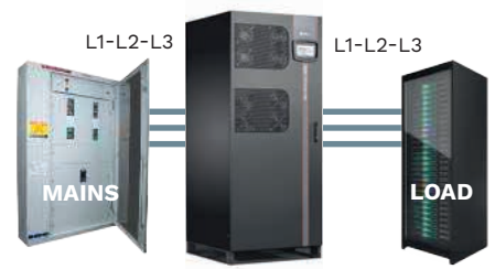
3-wire (L1-L2-L3) installation
